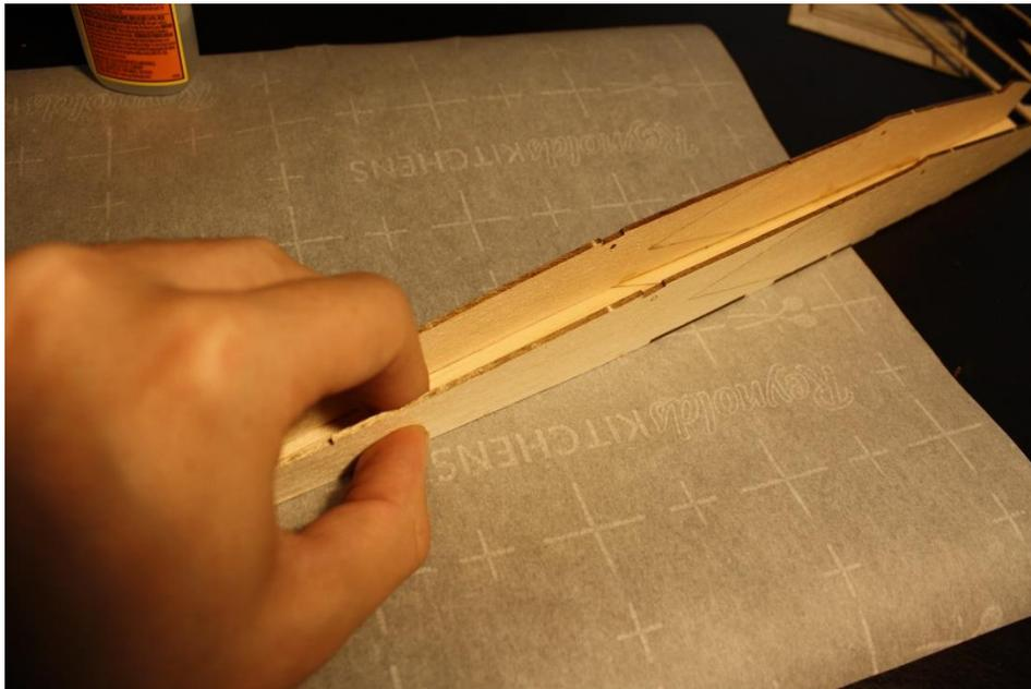
Now grab the top sheet. There are a few ways to glue this on. If you want, use medium or thick ca, apply glue on all of the mating surfaces, and put the top sheet on. I prefer a different method. Place the sheet on, hold it in place, and run some thin CA along the joints. It'll wick right in. I start at the back and work my way forward.
